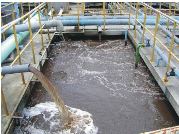
Installed on the municipal wastewater treatment plant
