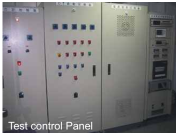
Test control Panel
