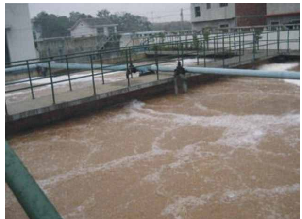
Real operation in sewage plant
