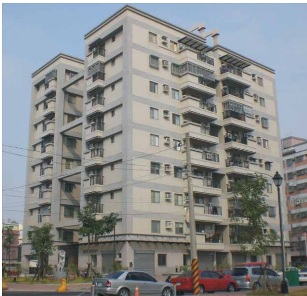
High building drainage system
