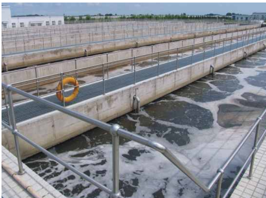
Industry wastewater aeration treatment
