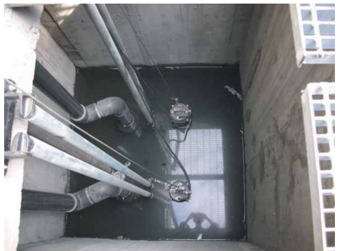
High building drainage system
