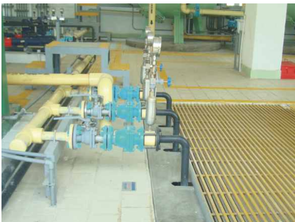
Installed on the wastewater treatment station
