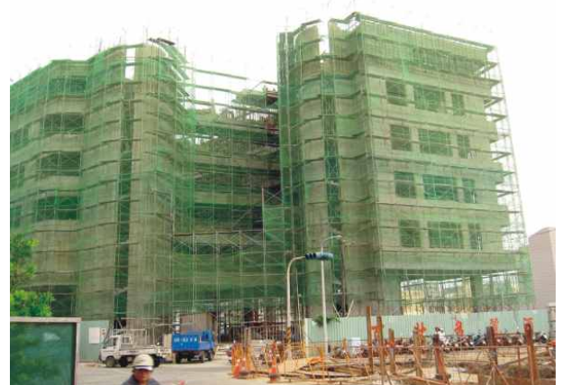
Building wastewater treatment system
