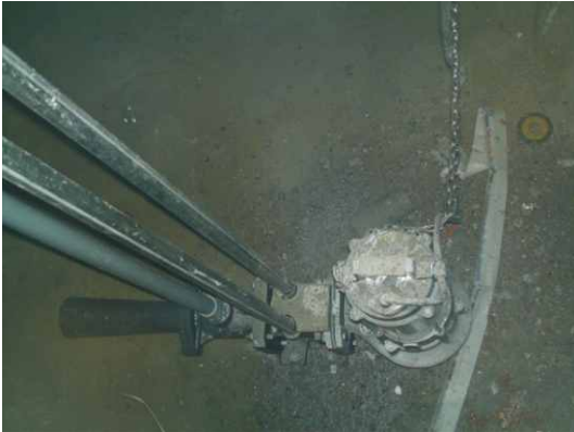
The real installation
