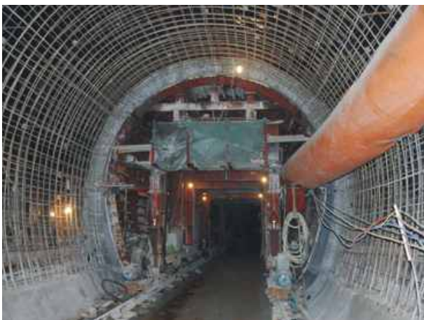
Applied in the drainage system of subway
