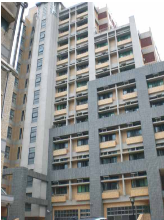
Mansion pumping system
