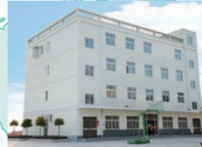
Qidong Head Office
